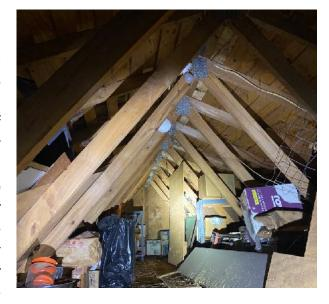
foundation and it is a non-load bearing part of the structure. Cracks were noticed on the garage ceiling. The cracks are due to minor deflection of the ceiling joists caused by over loading of the attic area. The load bearing capacity of the ceiling joists have not been affected.
